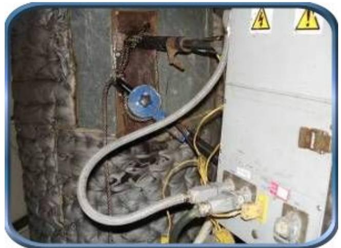
**Continuous measurement probe and sample collection probe, placed in the ME4 flue.**
